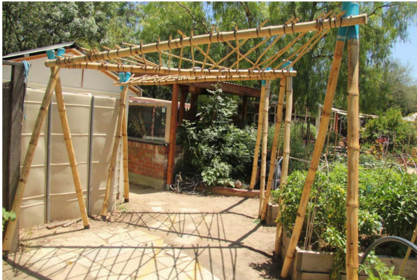
This small shade structure was built as part of a 2 day construction workshop for a community garden Peppertree Place in Coburg, Victoria. The structure is made from locally sourced Balcooa along with some imported bamboo stakes and tanking cane that were available in the garden.
