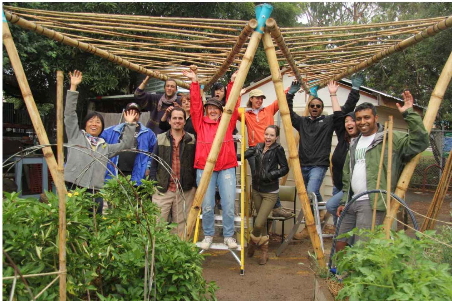
This small shade structure was built as part of a 2 day construction workshop for a community garden Peppertree Place in Coburg, Victoria. The structure is made from locally sourced Balcooa along with some imported bamboo stakes and tanking cane that were available in the garden.
